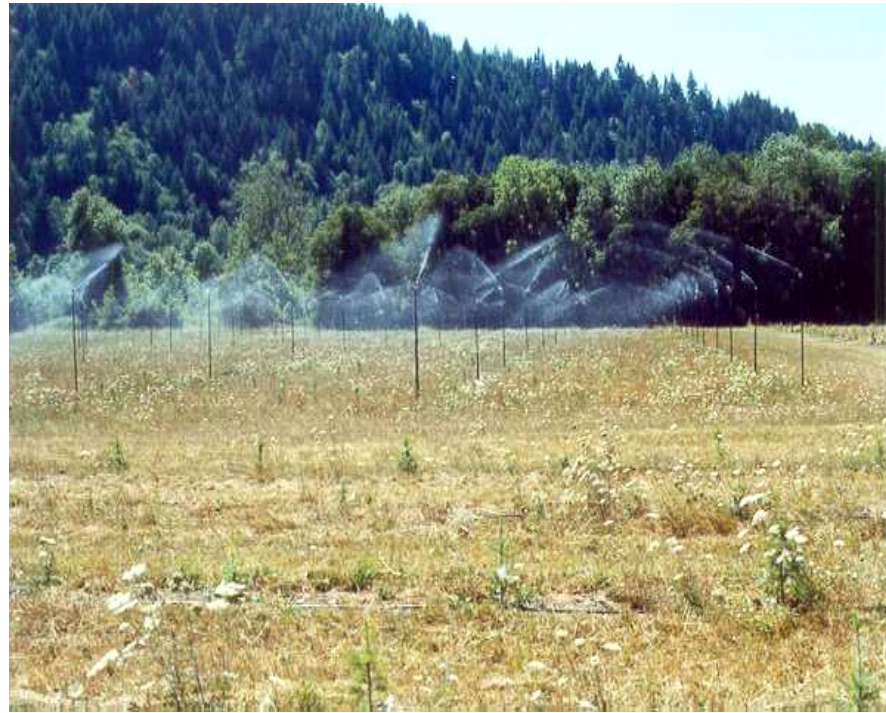
Figure 9. An overhead sprinkler system has been installed at the miniaturized seed orchard site.
